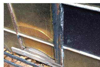
with steel reinforcements have rusted and deteriorated and need repair, repainting, and replacing
